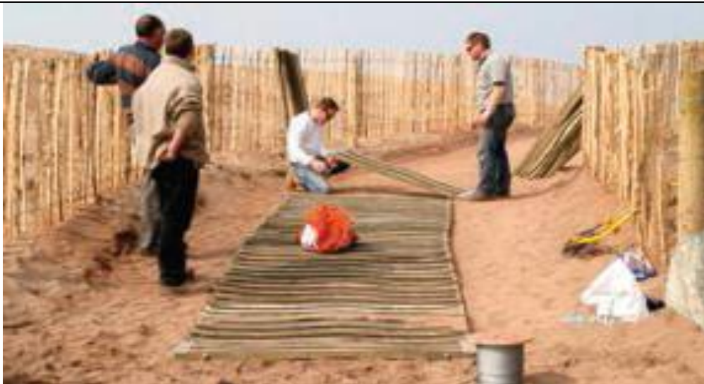
Figure 4.2.5: Establishment of a wooden pathway on a dune in the UK (From UK Sand Dune and Shingle Network Newsletter, July 2009).
